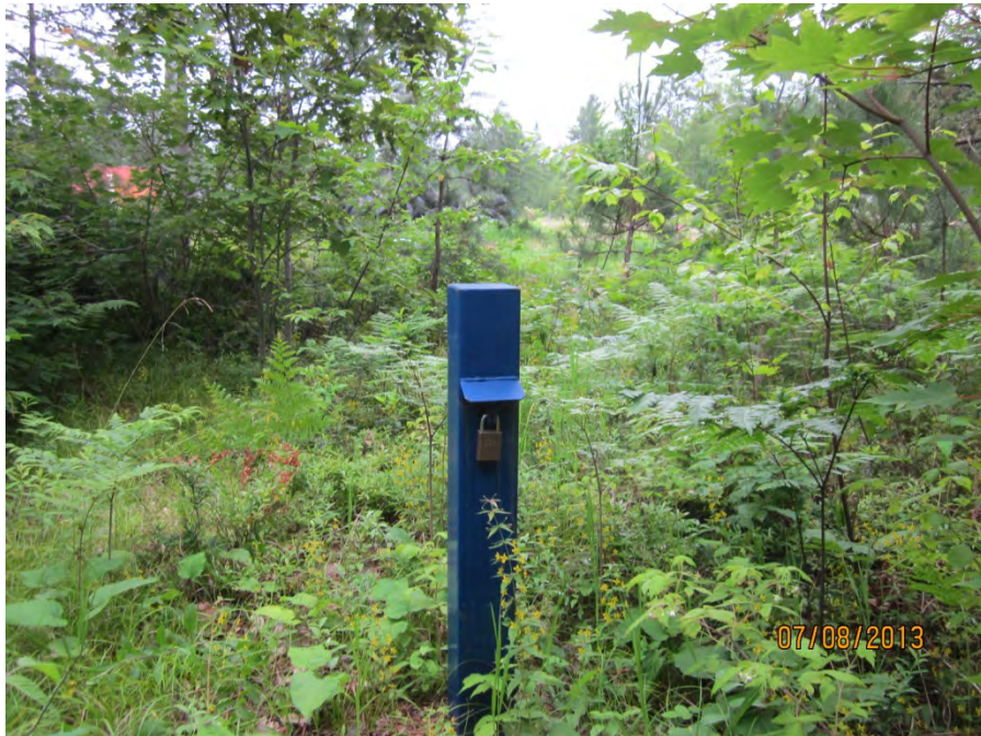
Photo 8 Groundwater monitoring wells BH7, July 2013
