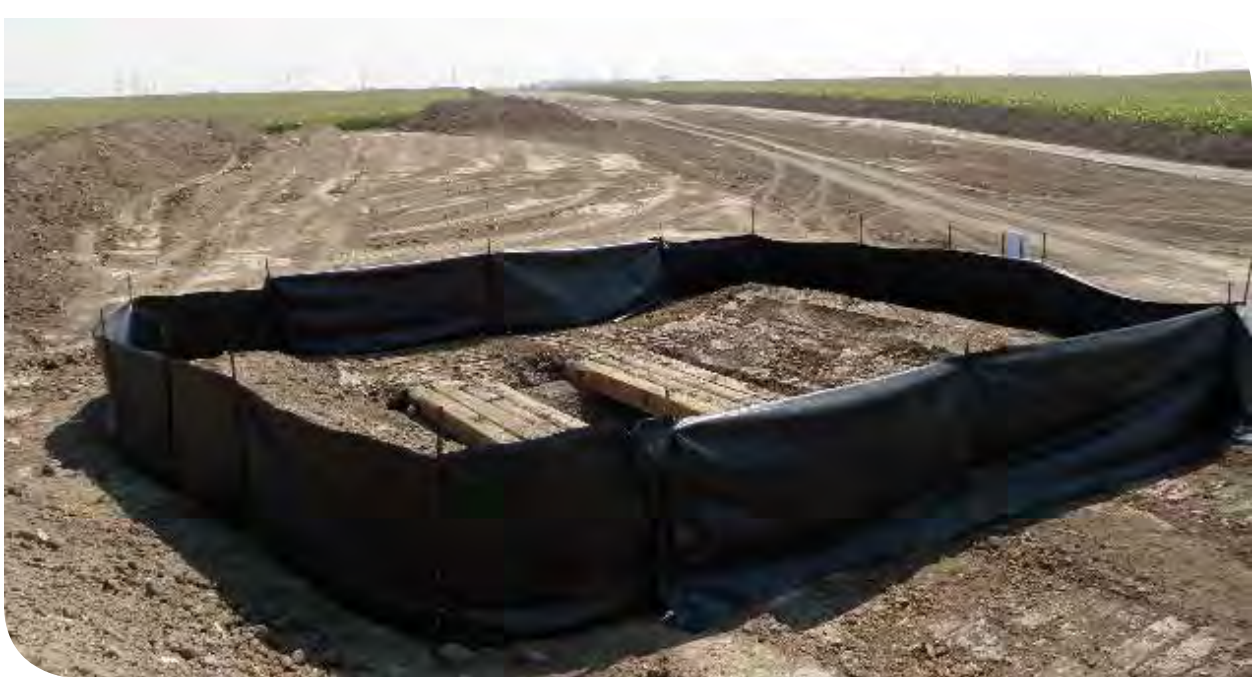
Cleaning station at construction site. Photo by: Mark Heaton, OMNR
