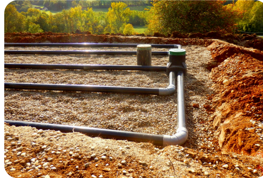
Septic system improvement
